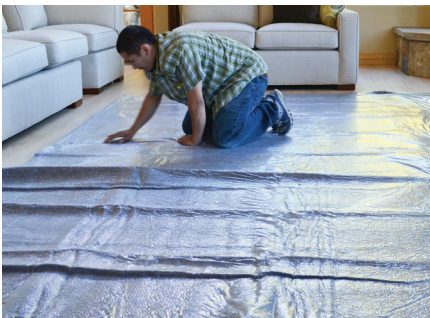
STEP FOUR using tape markers, stick pad to floor
