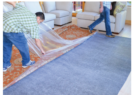
STEP SIX peel back top plastic layer revealing sticky top of pad
